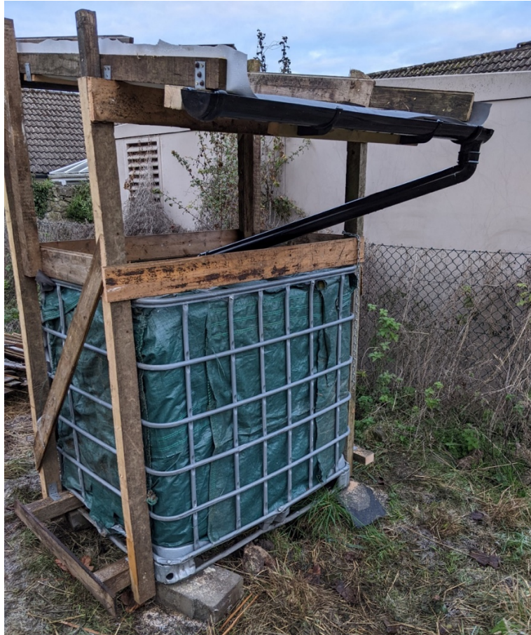
An IBC water collector installed to serve the Nursery
